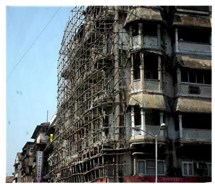
materials have been used to put scaffolding on the sides of the buildings for the workers to use. In Hong Kong the preference is for bamboo poles lashed together with cord. In Mumbai the scaffolding looks similar to that in Hong Kong, The poles are not bamboo but the trunks of a tree that appear to be about 3 inches in diameter. We took some photographs of the extensive scaffolding on several buildings.
